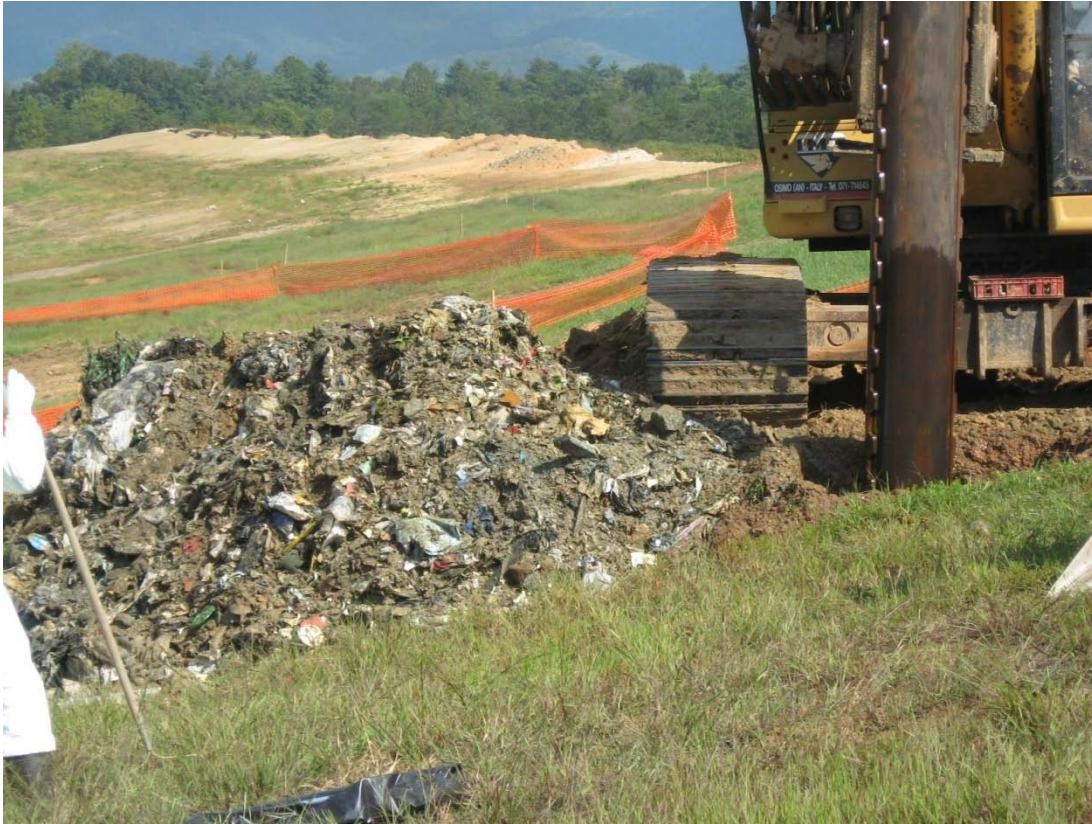
Figure 5-6 – Exhumed Waste from Drilling of Vertical Well 13
