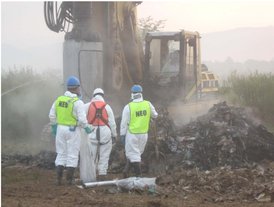
Figure 5-5 – Exhumed Waste from Drilling of Vertical Well 24
