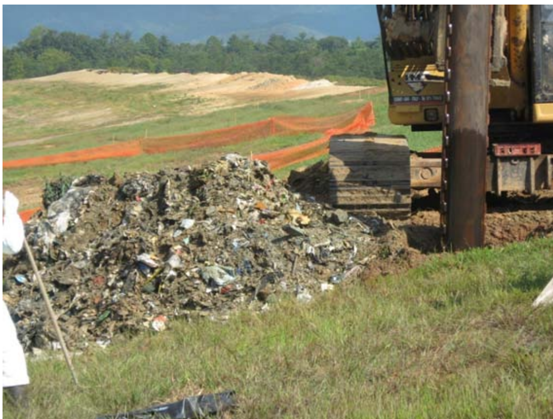
Figure 5-6 Exhumed Waste from Drilling of Vertical Well 13
