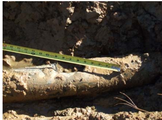
Cut Pipe to Replace
