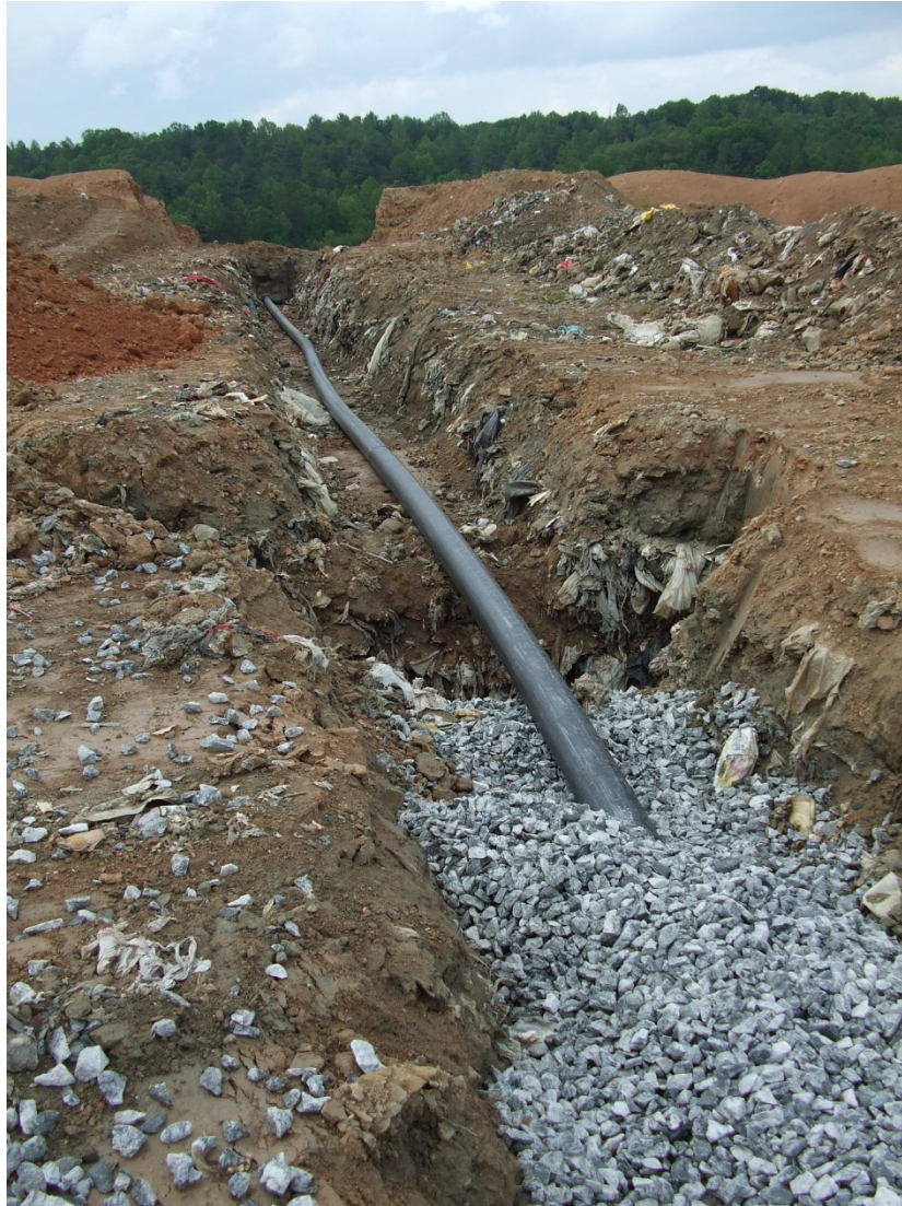
Figure 2-7 Horizontal Injection Trench Installation in Cell 6
