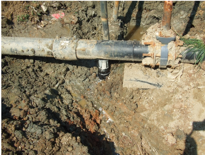
Replaced T-mold on HIT A
