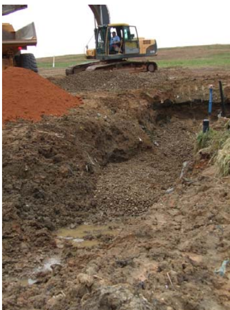
Continue Excavation, Drain Leachate Down and Place Gravel then Clay
