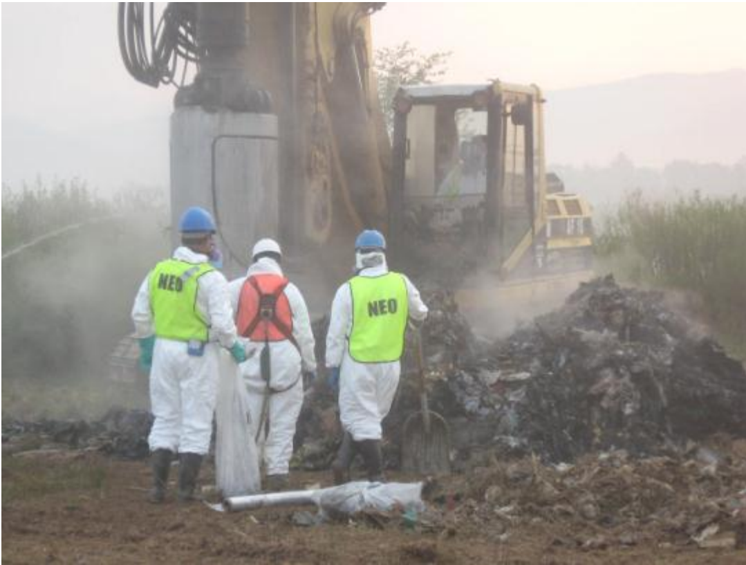
Figure 5-5 Exhumed Waste from Drilling of Vertical Well 24
