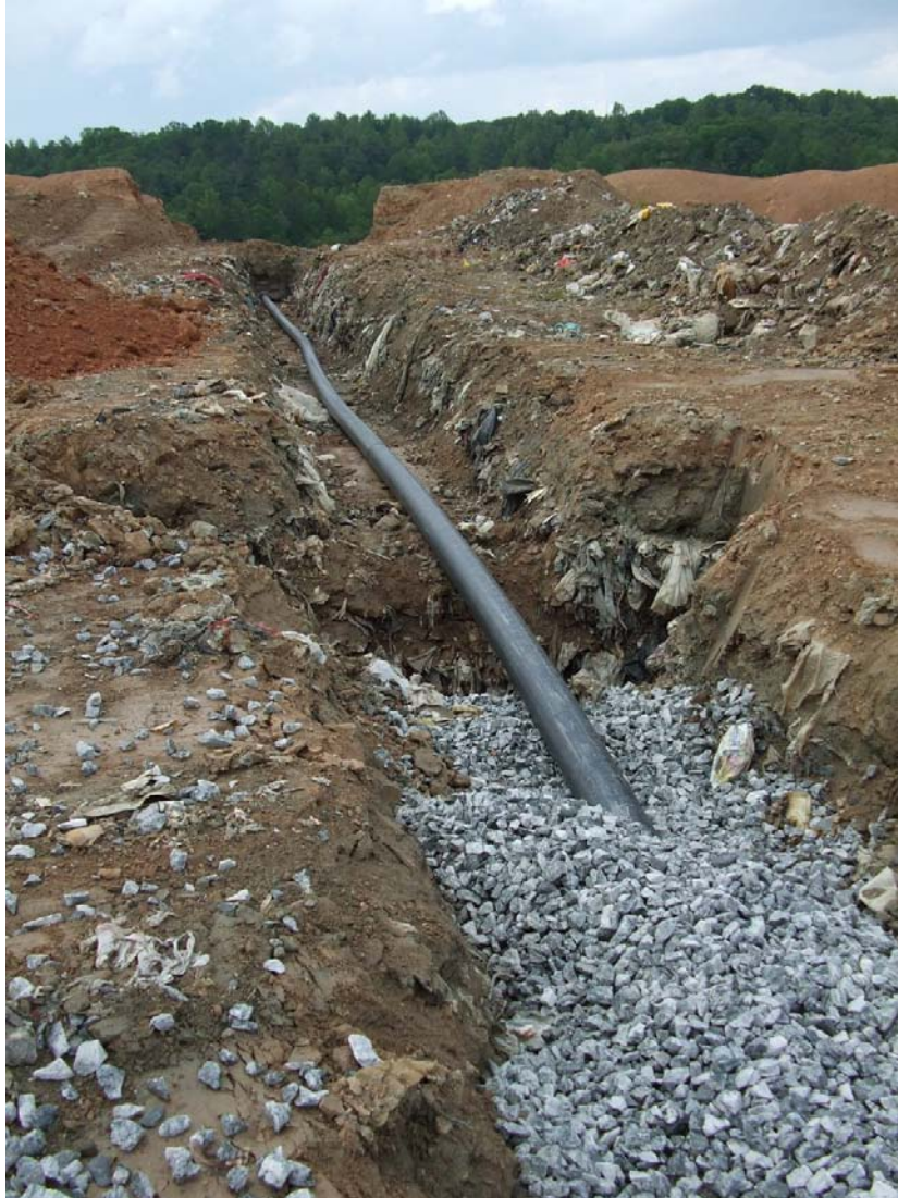
Figure 2-7 Horizontal Injection Trenches in Cell 6
