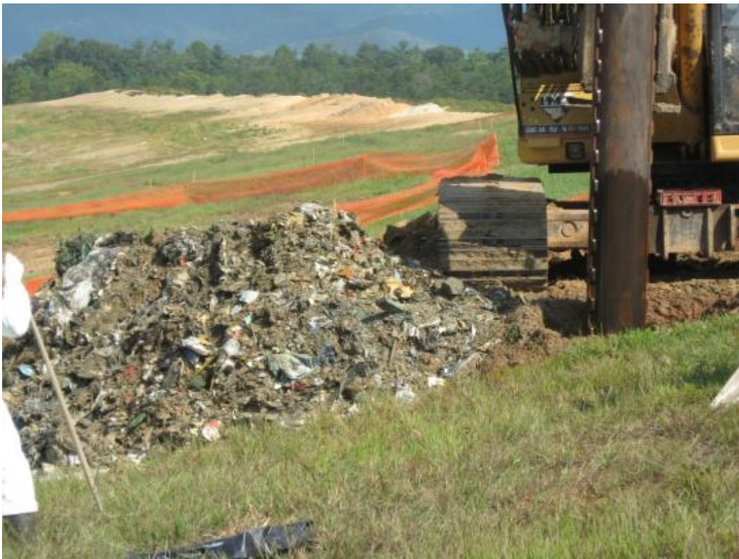
Figure 5-6 Exhumed Waste from Drilling of Vertical Well 13
