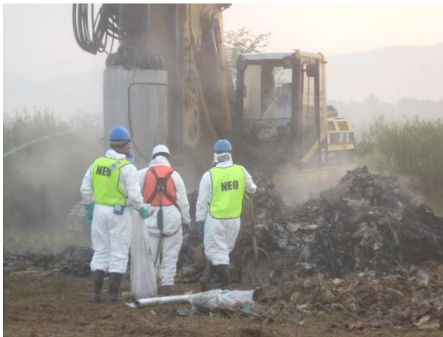
Figure 5-5 Exhumed Waste from Drilling of Vertical Well 24
