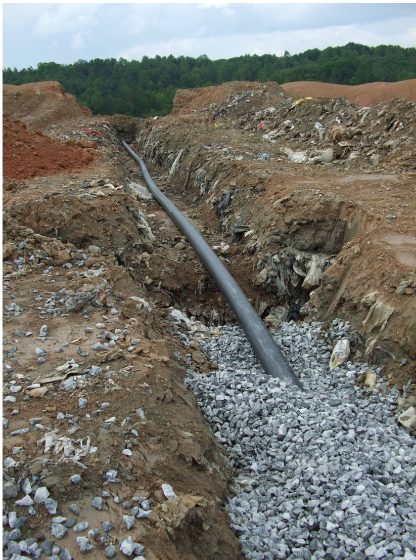
Figure 2-7 Horizontal Injection Trench Installation in Cell 6
