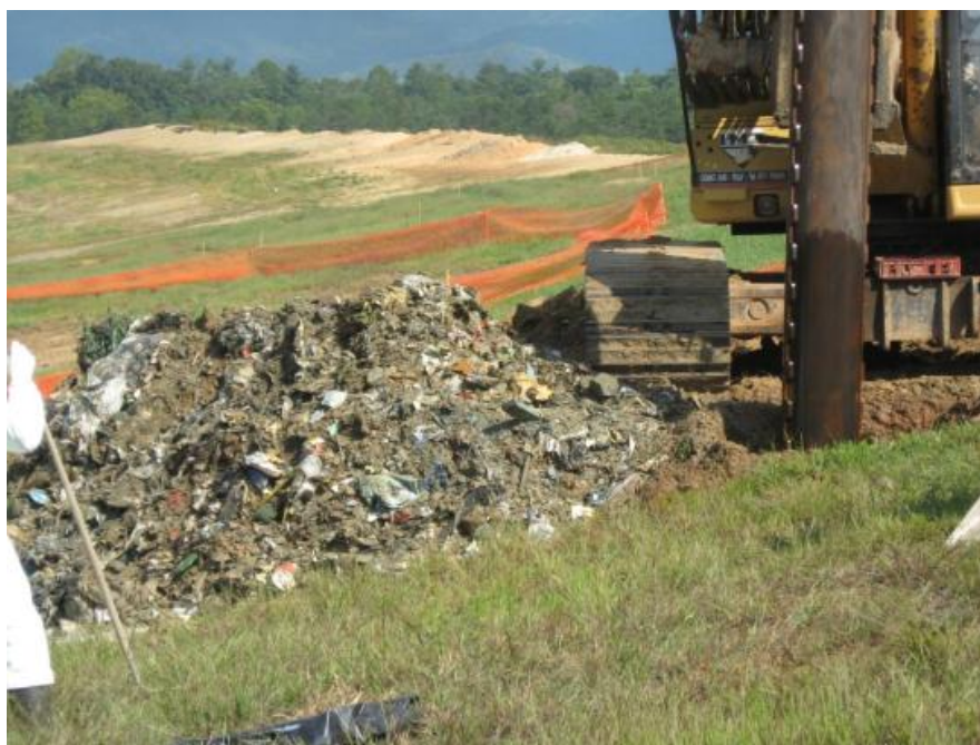
Figure 5-6 Exhumed Waste from Drilling of Vertical Well 13
