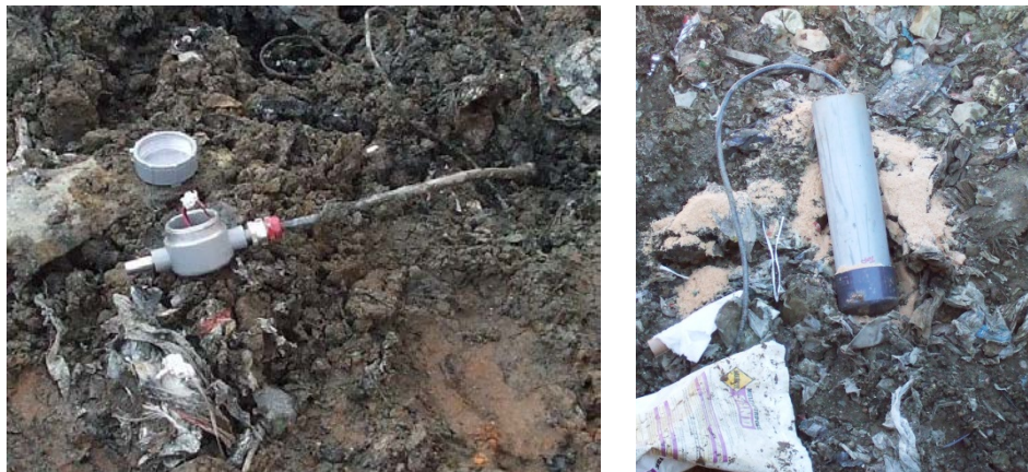
Figure 2-9 Installation of Thermocouples in Cell 6
