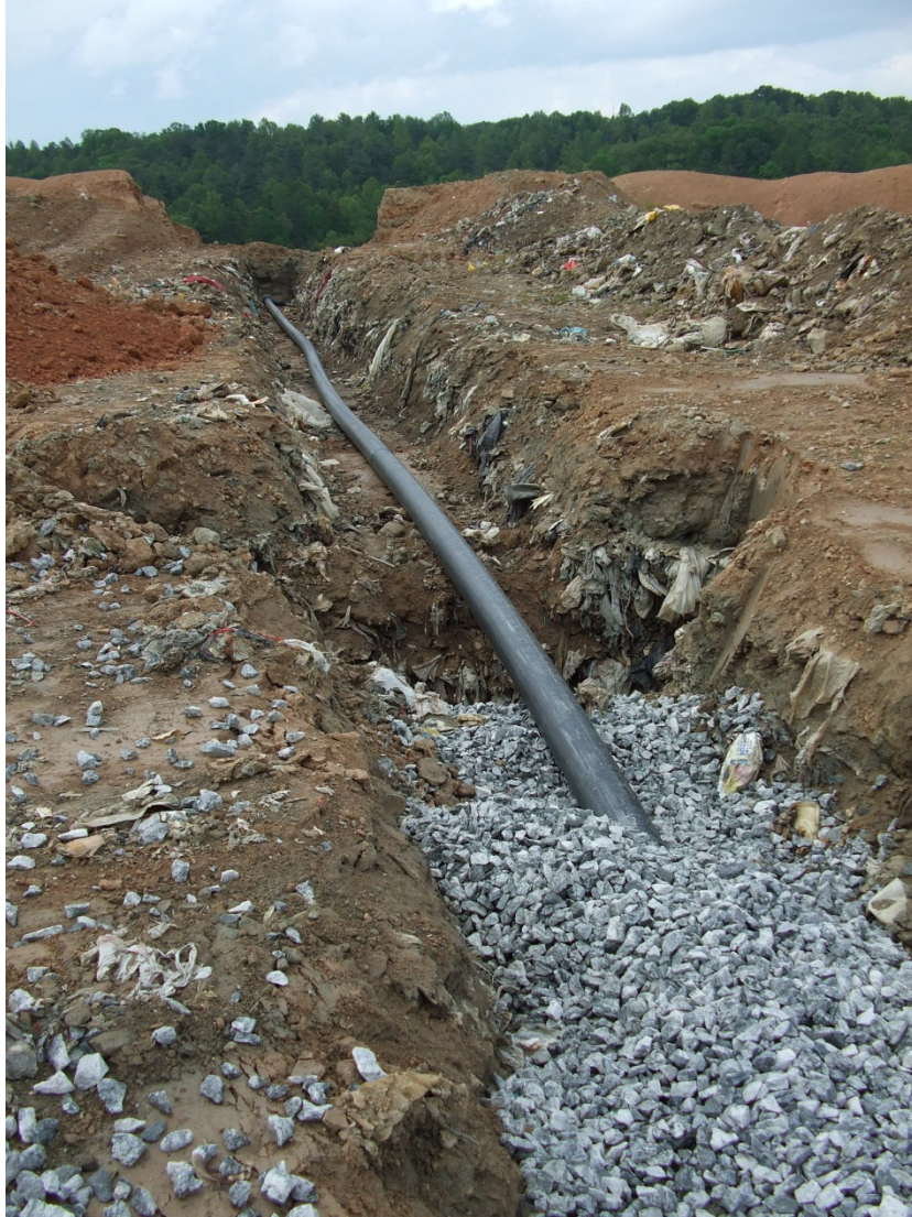
Figure 2-7 Horizontal Injection Trench Installation in Cell 6
