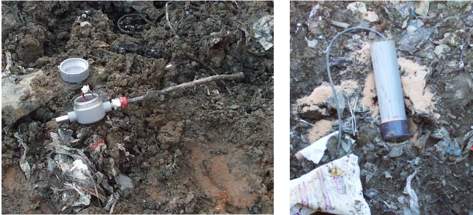
Figure 2-9 Installation of Thermocouples in Cell 6
