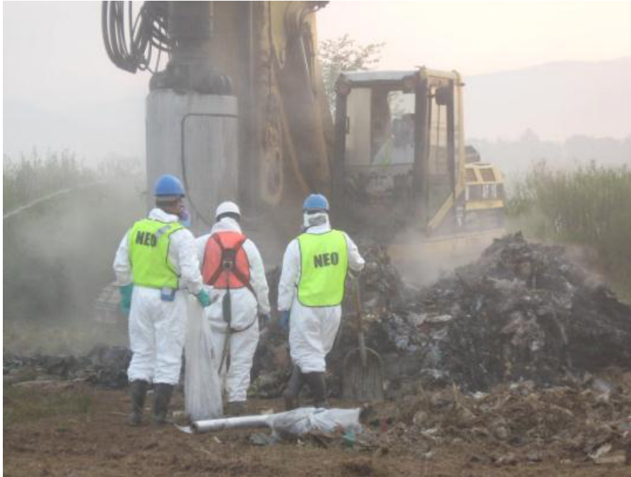
Figure 5-5 Exhumed Waste from Drilling of Vertical Well 24
