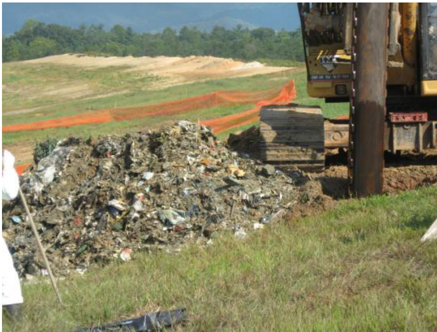
Figure 5-6 Exhumed Waste from Drilling of Vertical Well 13
