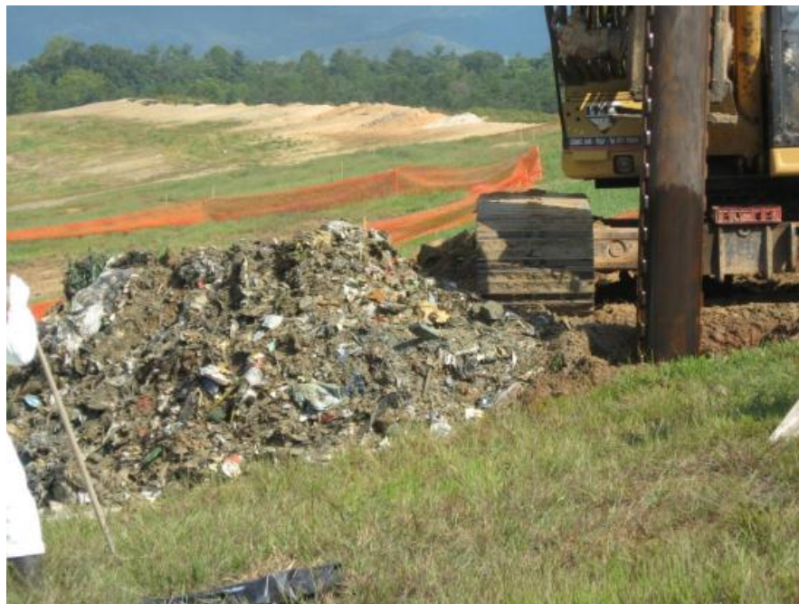
Figure 5-6 Exhumed Waste from Drilling of Vertical Well 13
