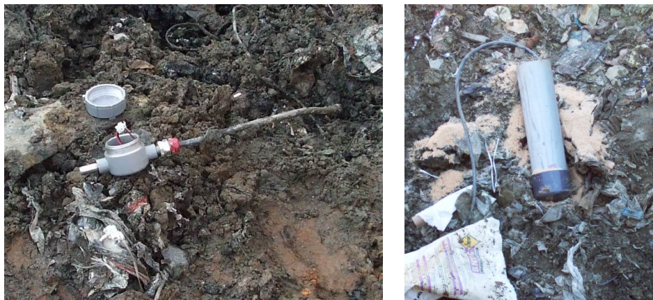
Figure 2-9 Installation of Thermocouples in Cell 6
