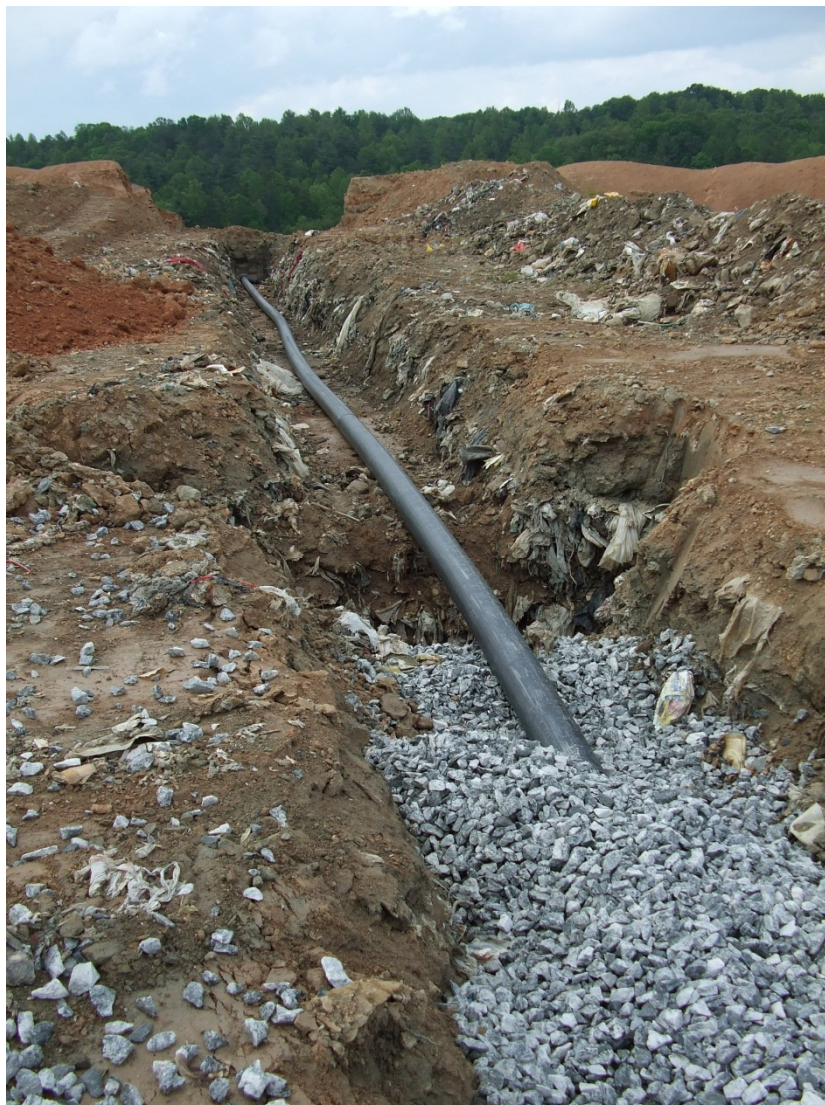
Figure 2-7 Horizontal Injection Trench Installation in Cell 6
