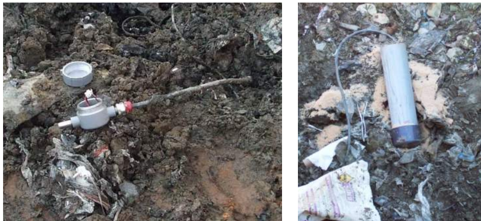
Figure 2-9 Installation of Thermocouples in Cell 6
