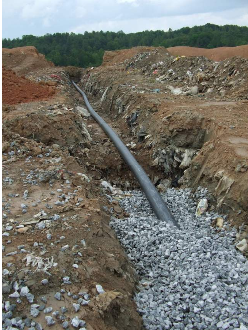
Figure 2-7 Horizontal Injection Trench Installation in Cell 6
