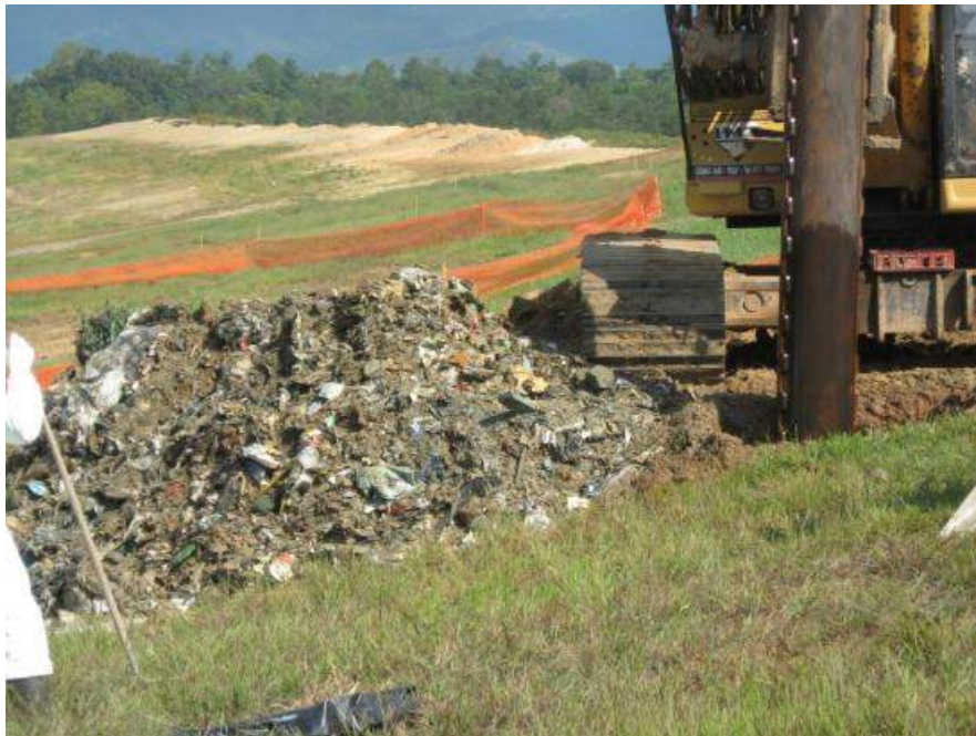
Figure 5-6 Exhumed Waste from Drilling of Vertical Well 13
