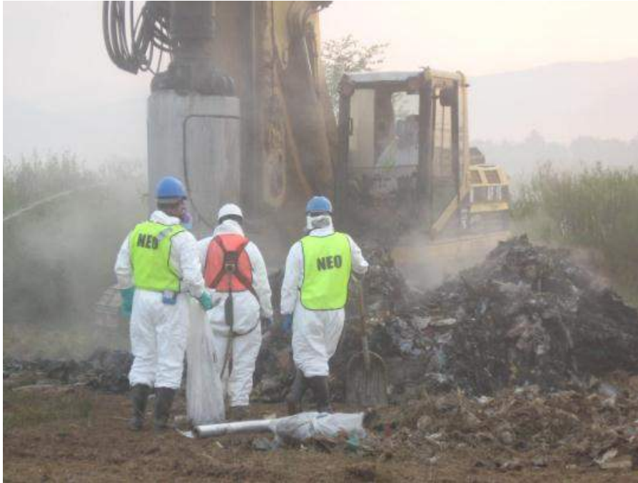
Figure 5-5 Exhumed Waste from Drilling of Vertical Well 24
