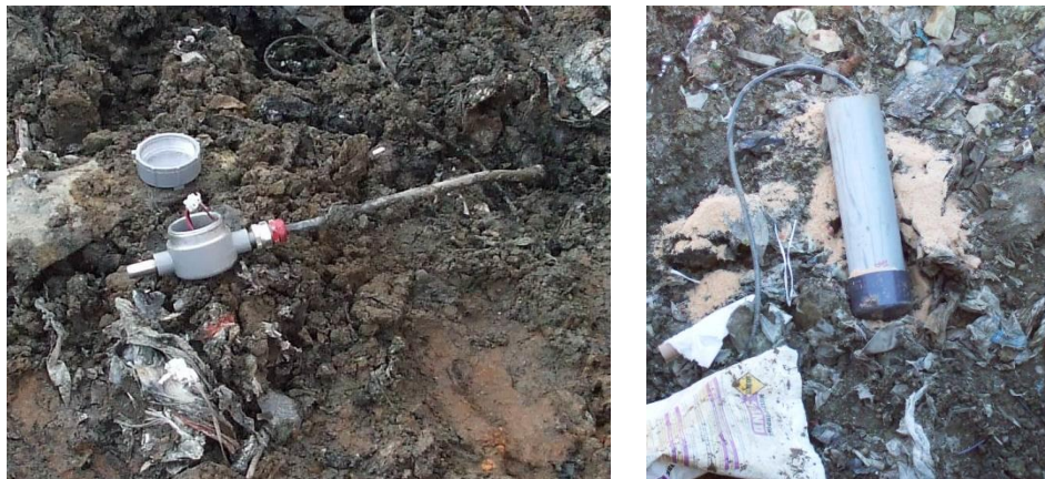
Figure 2-9 Installation of Thermocouples in Cell 6
