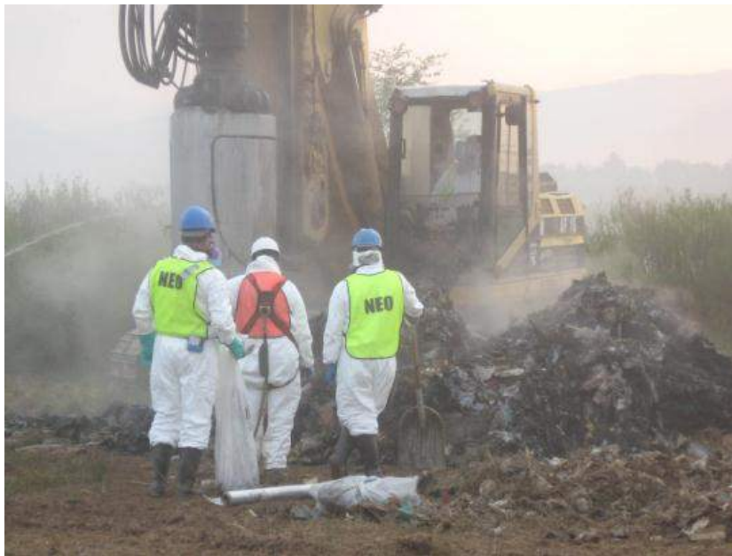
Figure 5-5 Exhumed Waste from Drilling of Vertical Well 24
