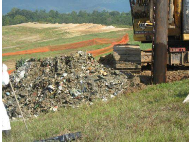
Figure 5-6 Exhumed Waste from Drilling of Vertical Well 13
