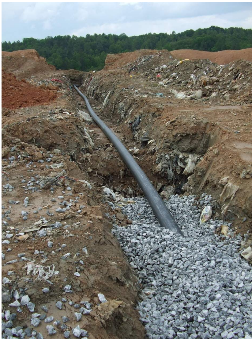
Figure 2-7 Horizontal Injection Trench Installation in Cell 6
