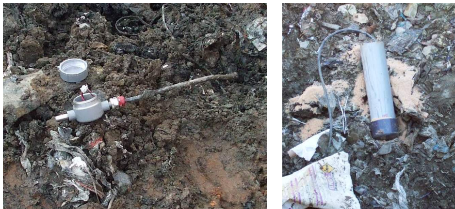
Figure 2-9 Installation of Thermocouples in Cell 6
