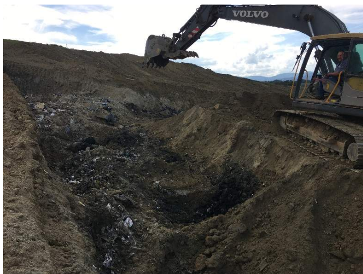
Figure ES-3: Excavation Around Gas/Leachate Line
