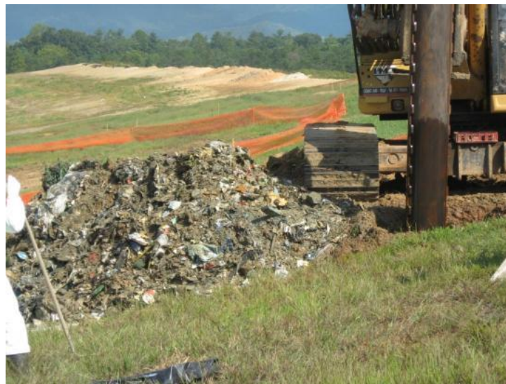
Figure 5-6 Exhumed Waste from Drilling of Vertical Well 13
