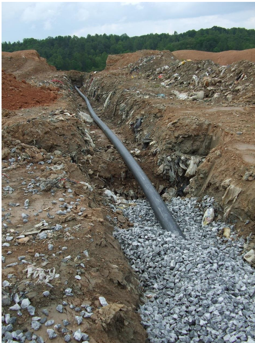
Figure 2-7 Horizontal Injection Trench Installation in Cell 6
