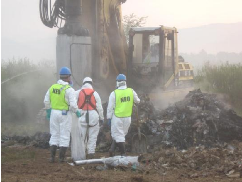
Figure 5-5 Exhumed Waste from Drilling of Vertical Well 24
