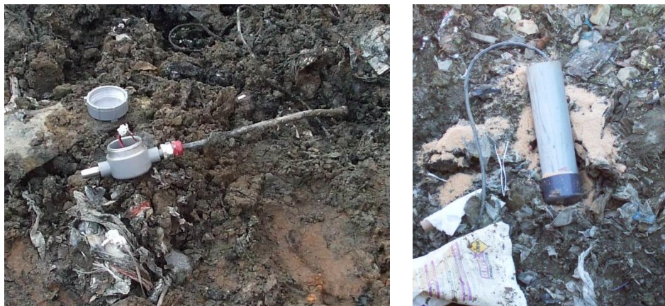
Figure 2-9 Installation of Thermocouples in Cell 6
