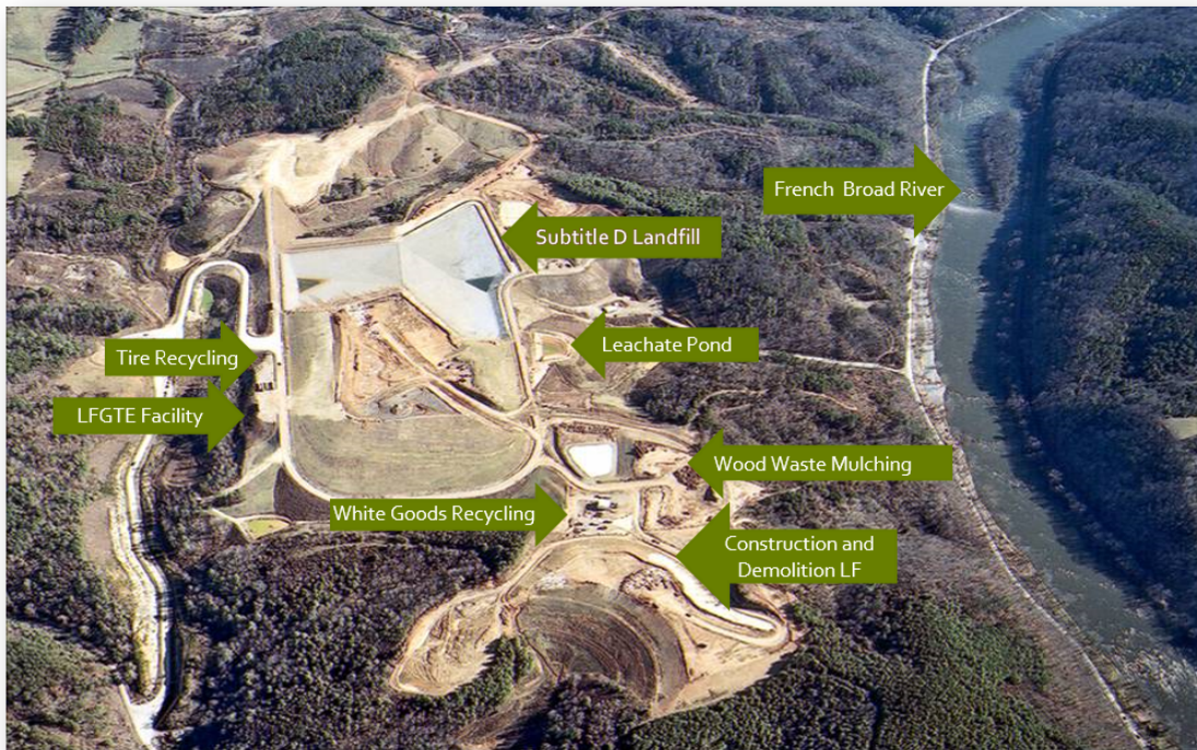
Figure 6. Buncombe County Solid Waste Management Facility
