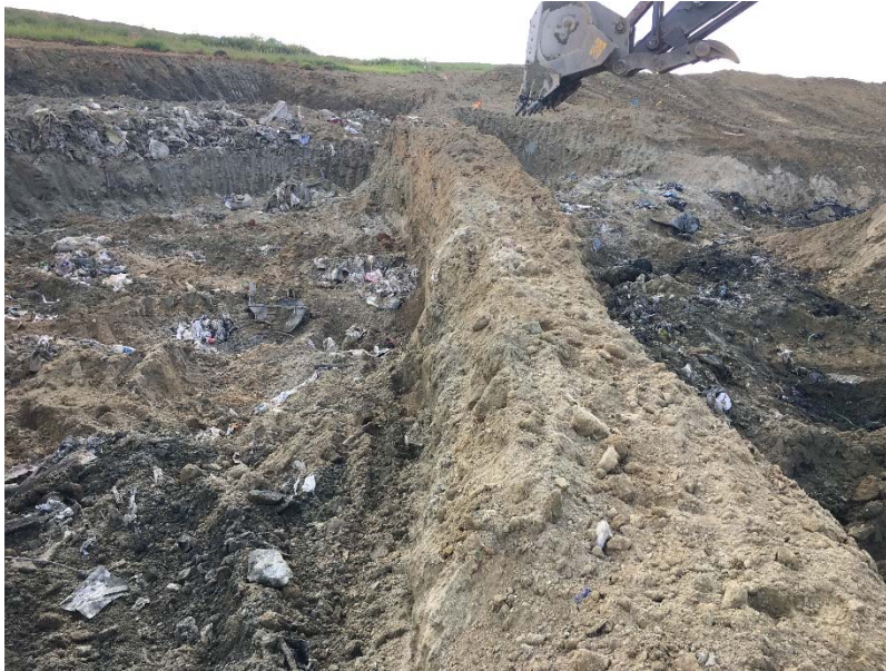
Figure 5. Excavation around Gas/Leachate Lines
