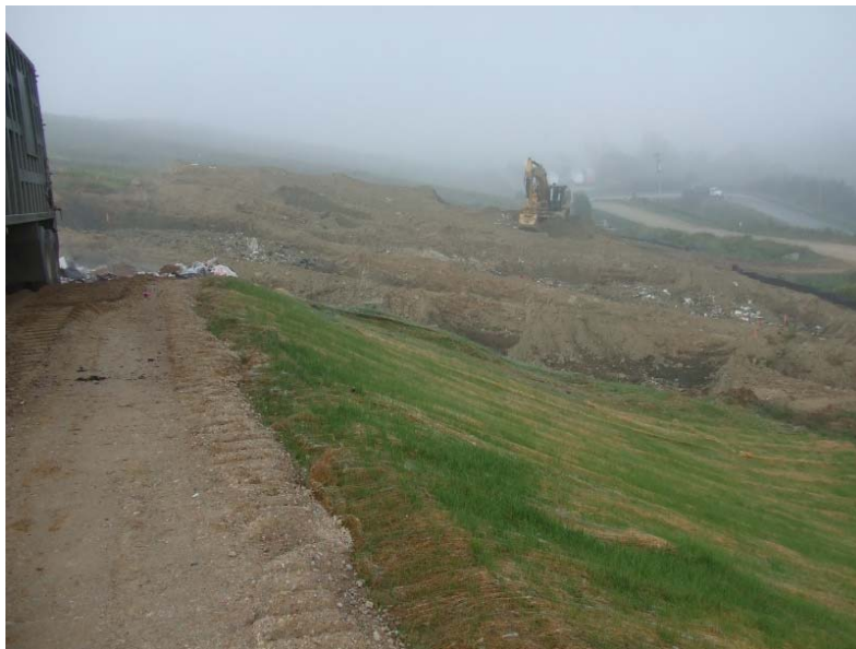
Figure 2. Access road to side slope disposal area
