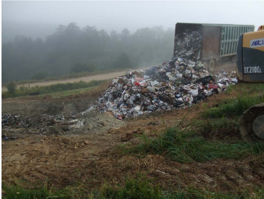
Figure 3. Side slope Waste Placement
