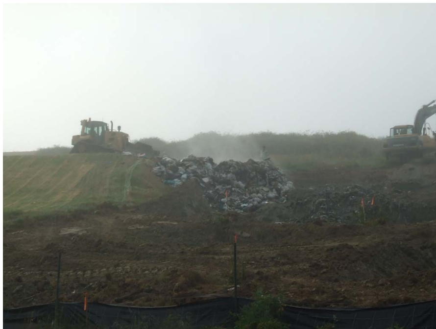
Figure 4. Waste Placement into sideslope disposal area
